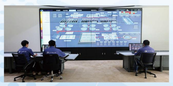
has an online monitoring system which monitors inlet and outlet water quality for 24 hours per day. Monitoring data are transferred simultaneously to municipal and provincial-level comprehensive monitoring and management platforms on pollution sources. Wastewater after treatment meets requirements as set out in the Discharge Standard of Pollutants for Municipal Wastewater Treatment Plant (《城鎮污水處理廠污染物排放標準》(GB18918-2002)).
